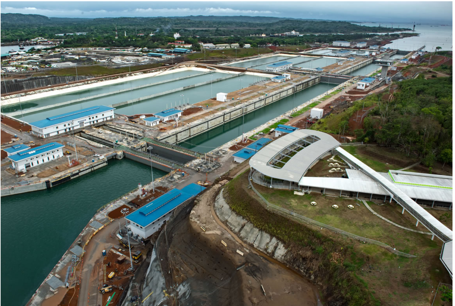
Water saving basins at the Agua Clara Locks, Atlantic side.
